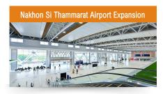
**Project:** The expansion adds a 30,600-square-meter terminal with eight gates and extends the runway to 2,990 x 45 meters, increasing capacity for four million passengers and larger aircraft.
